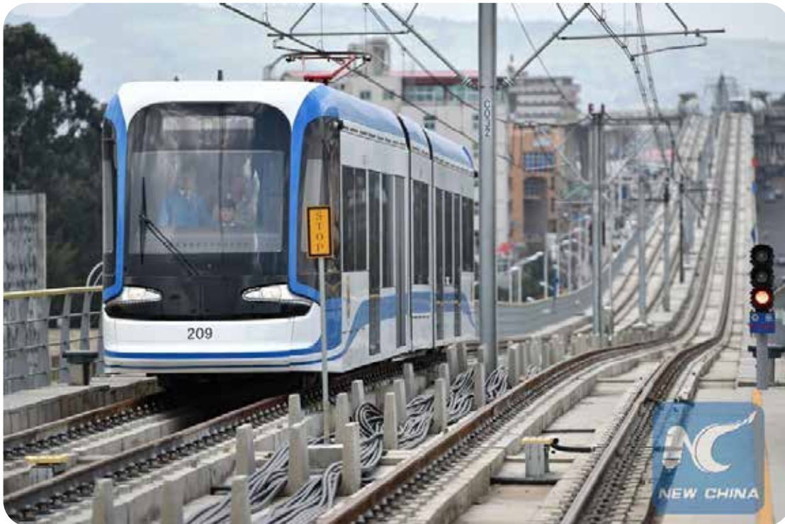
Train operating on the light rail in Addis Ababa, Ethiopia. (Photo: Xinhua/Sun Ruibo, 20 September 2015)
