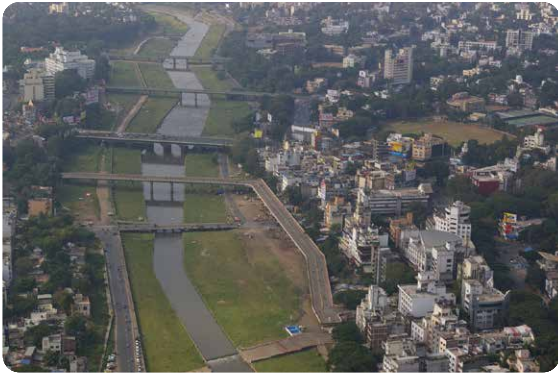
Pune, Bridges are improving urban mobility and connectivity (Photo: Mangesh Dighe, Environmental Officer, Pune Municipal Corporation)
