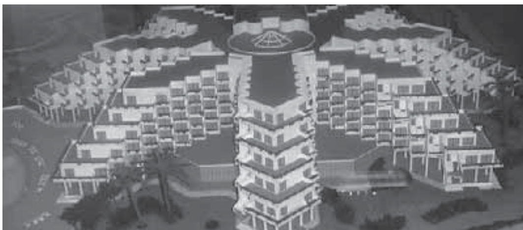
Fig. 7. Hotel Meliá Varadero. Its petal shape takes advantage of the various directions of the wind for natural cooling. The central atrium acts as a "chimney" expelling the warm air. The walls around the atrium are covered by hanging vegetation to absorb heat in the evapotranspiration process. Fresh air passes through the doors of the petals, resulting in comfortable temperatures during most of the year. (Source: CIGET)
