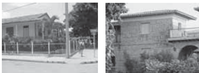
Fig. 5. Typical construction dating from the period 1910–1945
